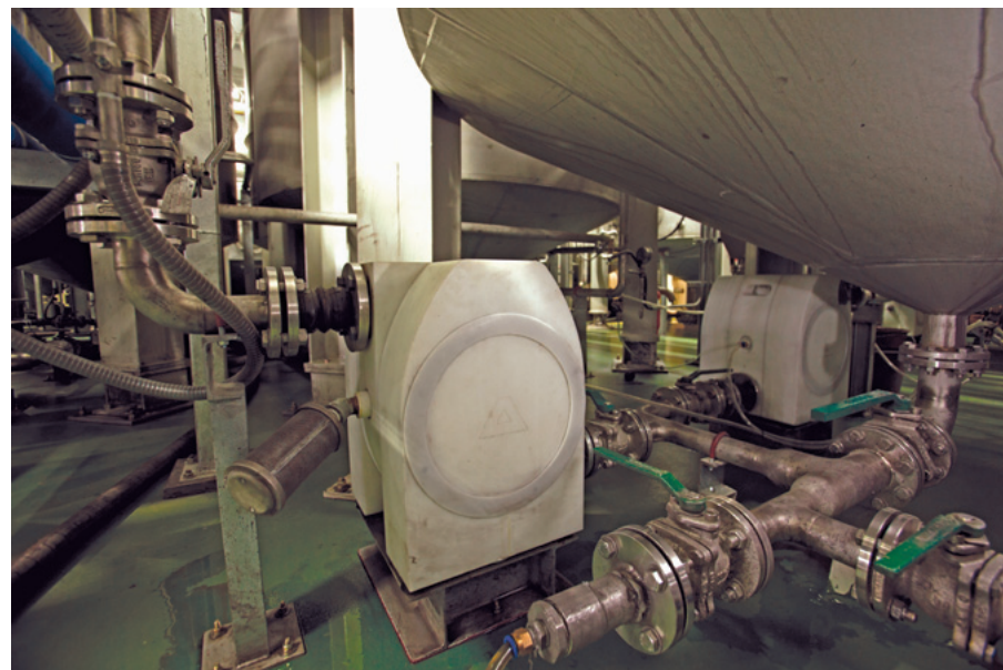
Application photo of an E-Series pump installed in a slurry application.
